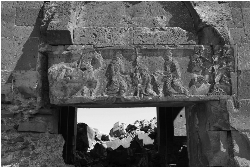
FIGURE 12.1. The church of Mren, ca. 638–640, north façade portal (Kars region, modern eastern Turkey). Photo: Christina Maranci.
